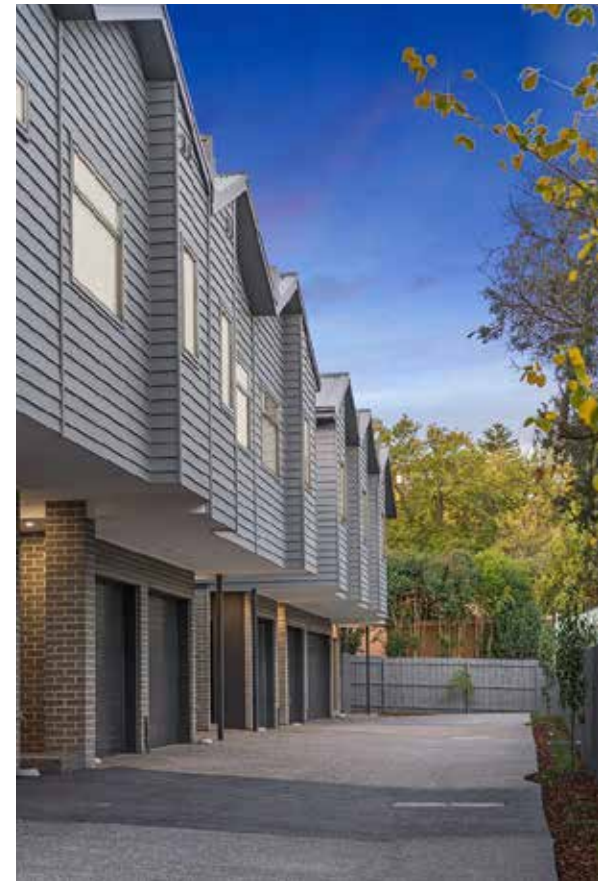
Figure 44. Emerging built form in the residential precinct
